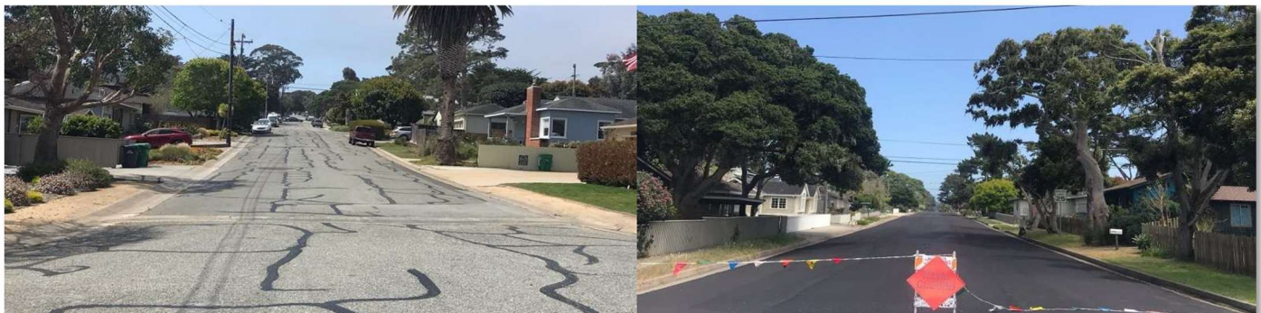
Crack and Slurry Seal
