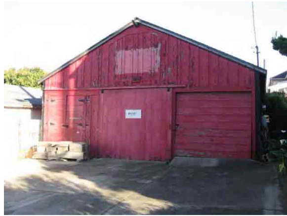
Former stable behind 122 18 th Street (facing 19 th Street)
