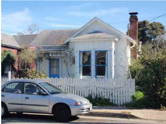
Gable-and-wing cottage, 229 19 th Street (1893)
