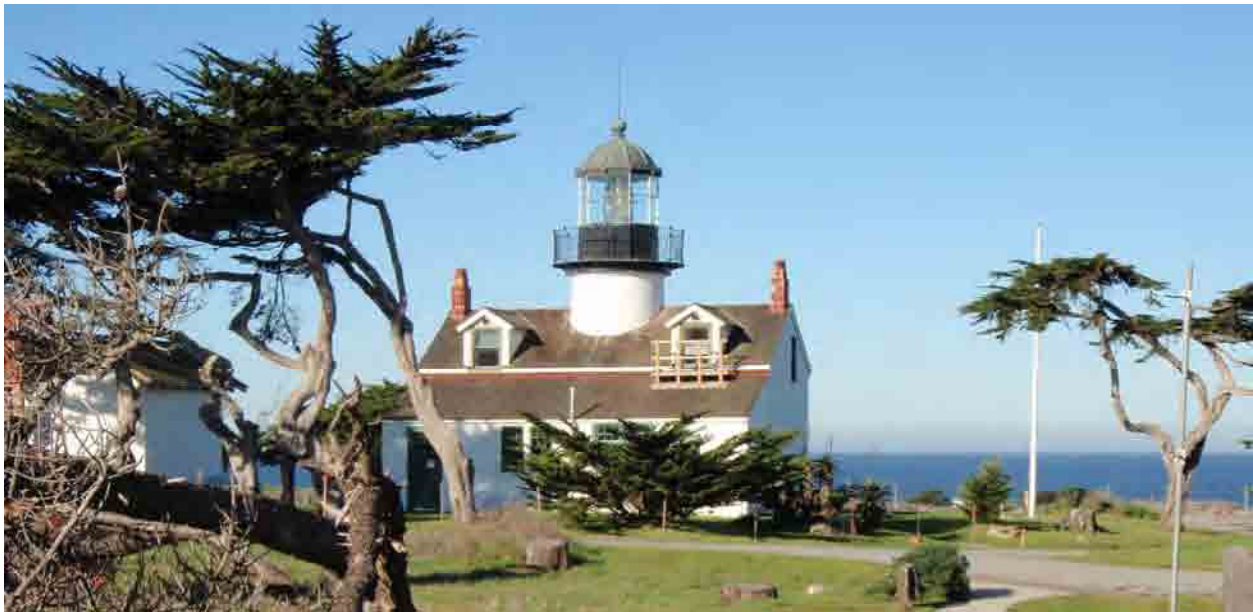
The Point Pinos Lighthouse, constructed in 1854, is the only extant resource from this period.
