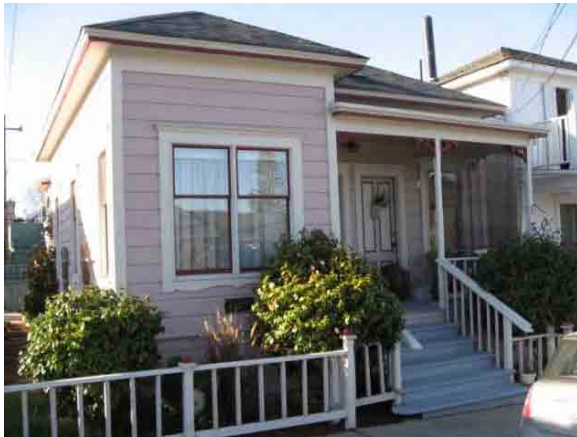
This vernacular duplex at 124 18 th Street (1887) employs few decorative elements
