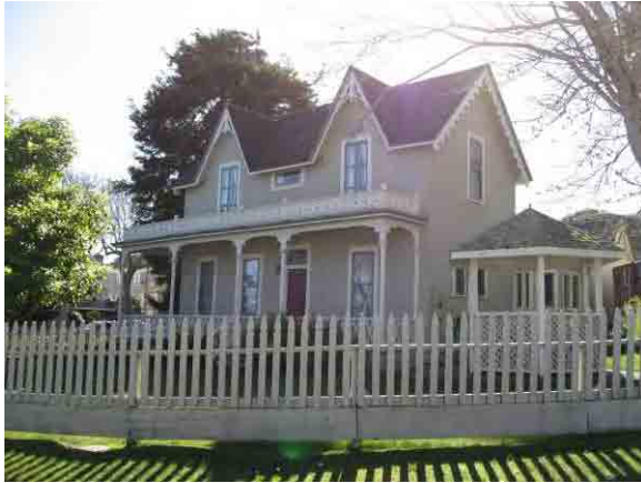
Gothic Revival-style house at 129 Pacific Avenue (1884)
