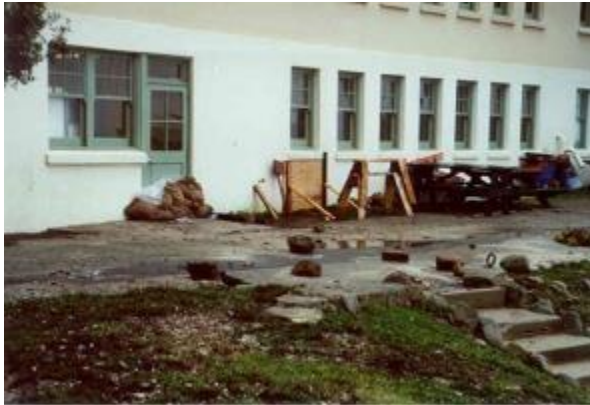
Damage from strong storm surges at Hopkins Marine Station. Photo Credit - Gary Griggs, Ph.D., presentation: Sea-Level Rise, Shifting Shorelines and El Niño 11/11/15
