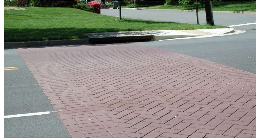
Crosswalk with the look of interlocking brick pavers. (Image credit: alternative-paving.com.)
