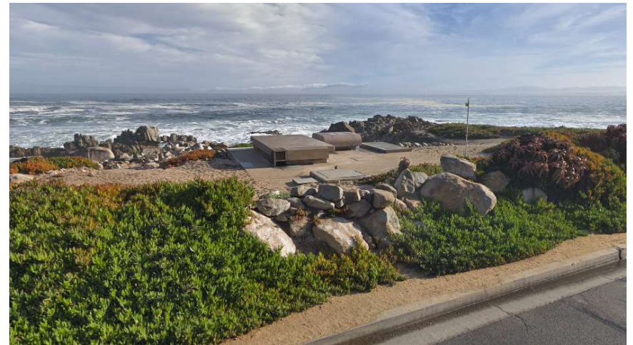
The pump station at its current location, between Esplanade Park and Coral Street. (Image credit: Google Street View.)
