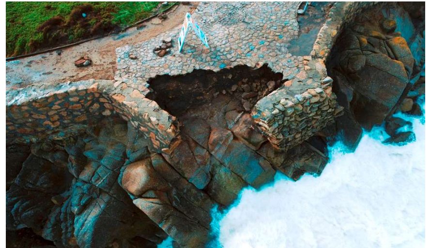
Overhead view of the collapsed section of seawall across from 701 Ocean View Boulevard.
