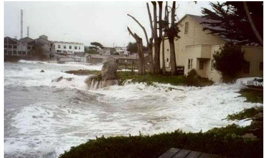
Waves and surge impacting buildings on the protected shore of Hopkins Marine Station, January 11, 2001. (Image credit: Hopkins Marine Station.)
