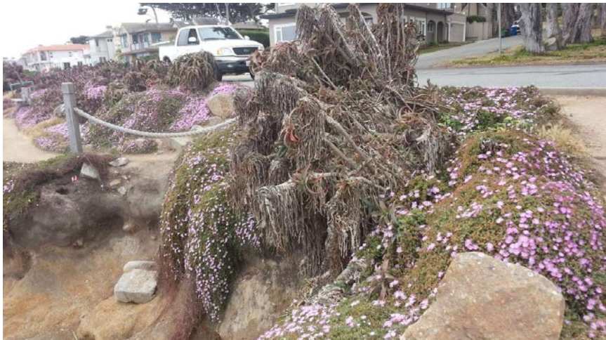
Bluff erosion across from Esplanade Park. (Image credit: Haro, Kasunich and Associates.)
