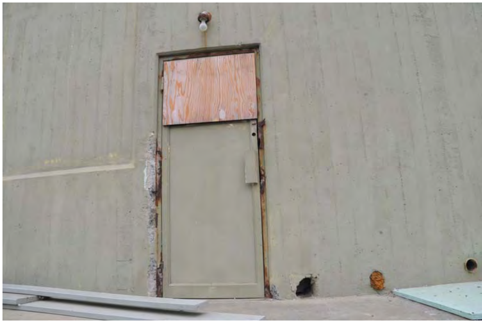
E-11 View of a door, illustrating moderate to severe corrosion on the door frame.
