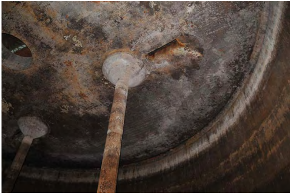
I-5 View of a portion of the roof, illustrating random corrosion on the roof and column.
