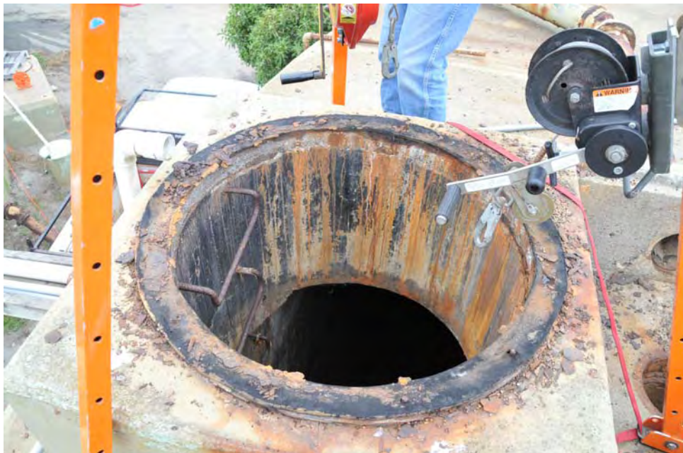
E-10 View of the roof hatch, illustrating staining and rust scale.
