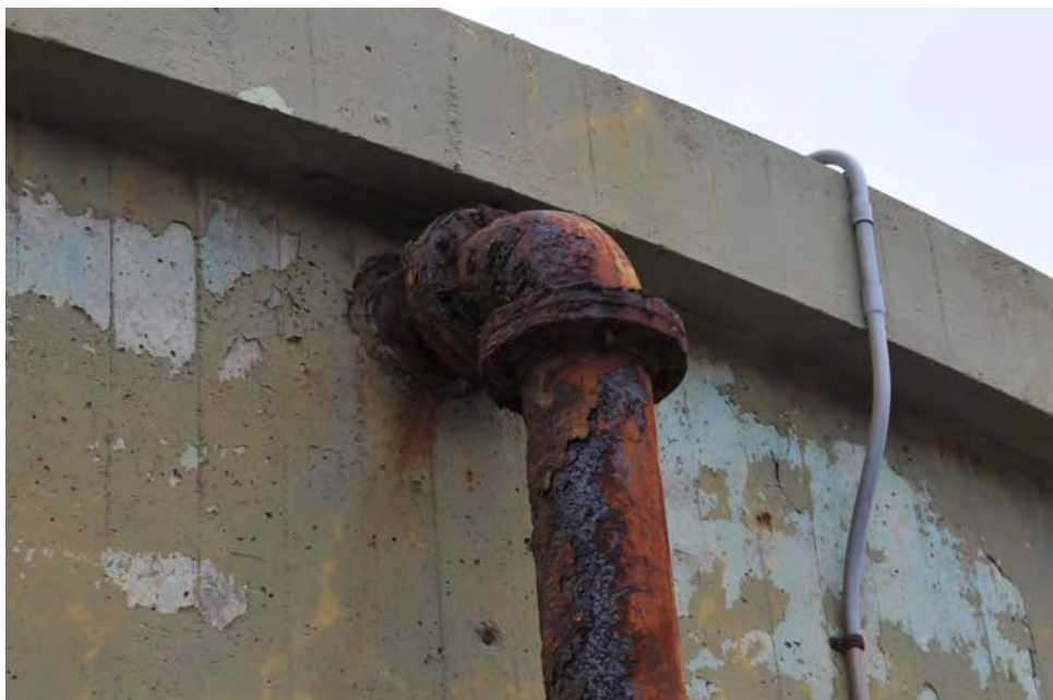
E-16 View of the overflow, illustrating severe corrosion of the piping and delamination of the adjacent paint system.
