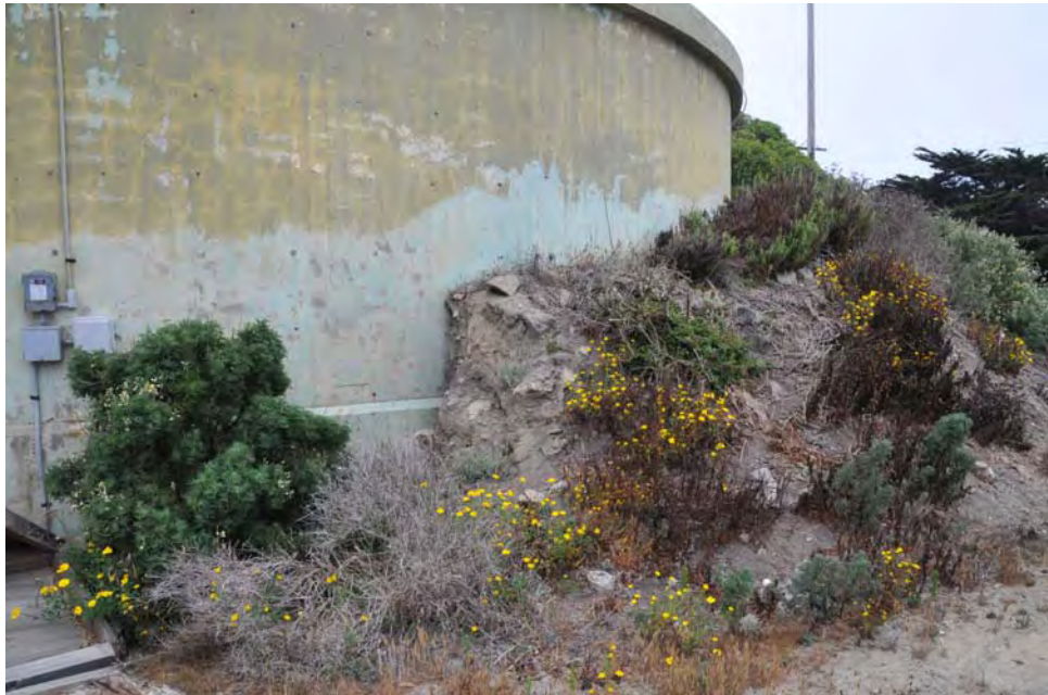
E-18 View of a portion of the wall, illustrating a dirt berm that has been pushed up against the wall.
