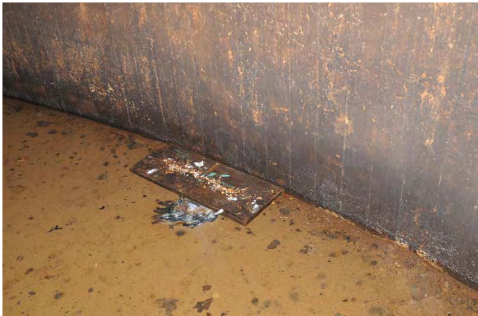
I-28 View of the wall to bottom transition, illustrating residue and staining of the concrete surfaces and dirt and debris in the water.
