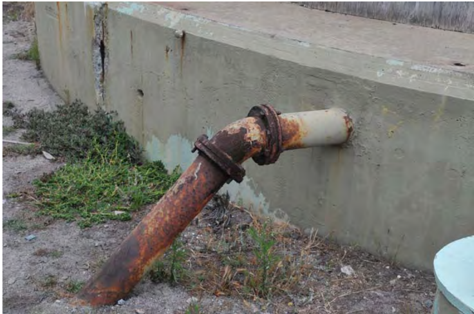
E-18 View of a penetration, illustrating moderate to severe corrosion.
