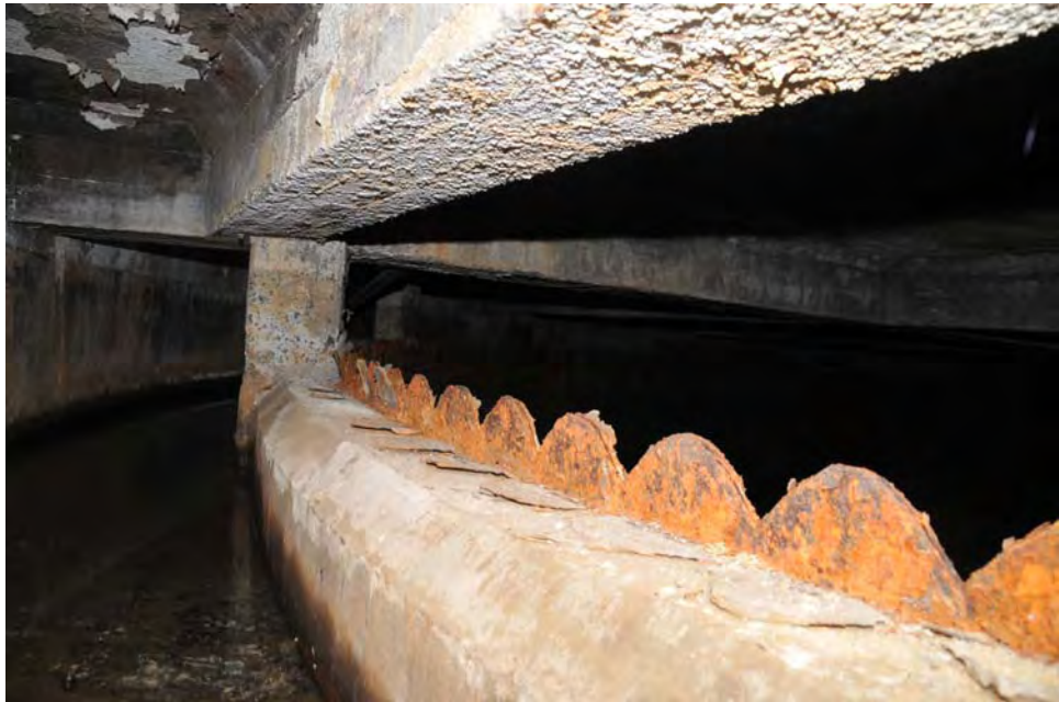
I-15 View of the interior effluent weir surfaces, illustrating severe corrosion on the weirs and delamination of the adjacent concrete roof surfaces.
