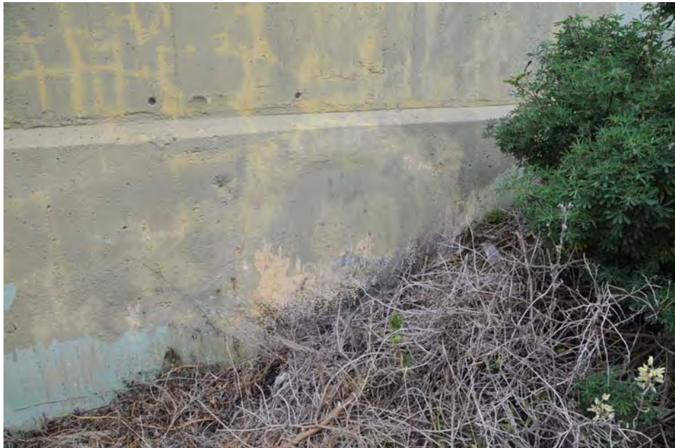
E-21 View of a portion of the wall, illustrating a penetration that has been filled and patched.
