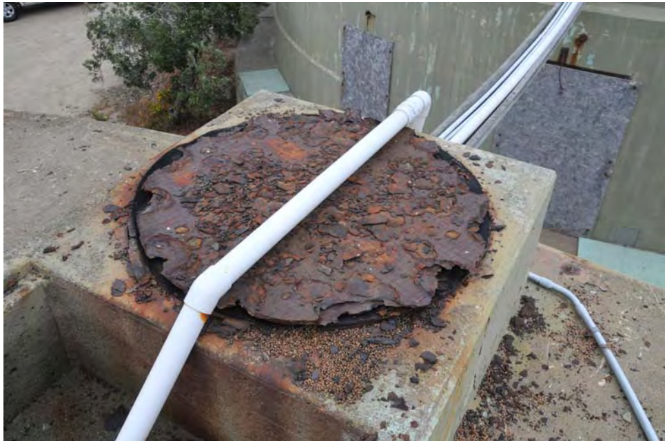
E-9 View of the roof hatch, illustrating severe corrosion of the cover.
