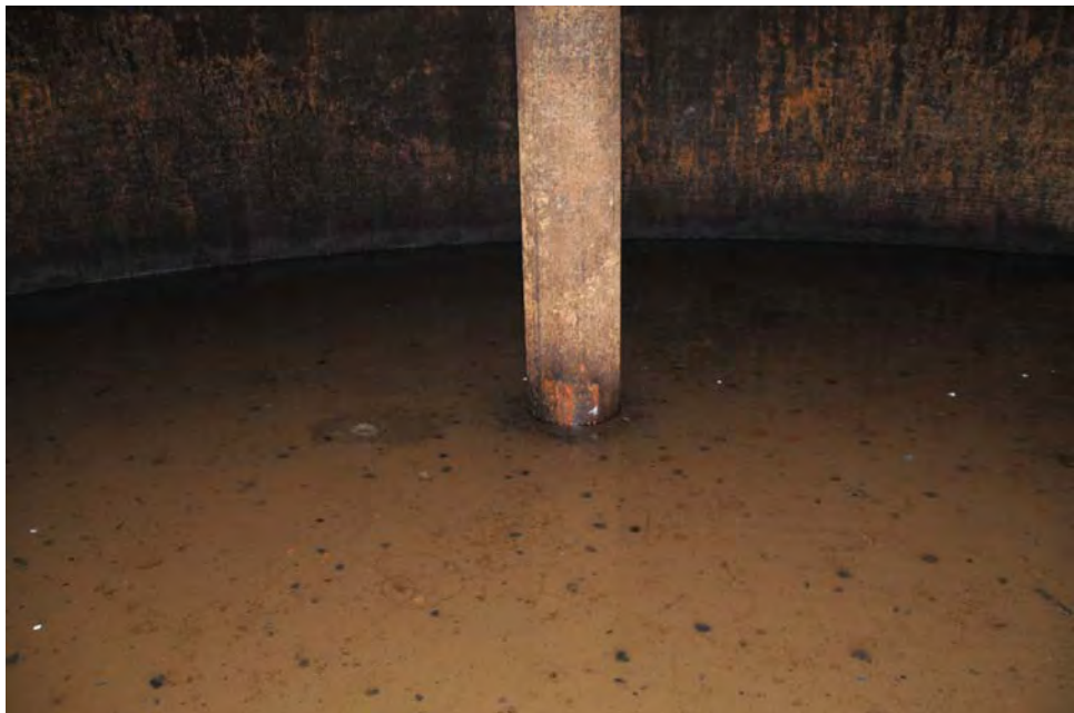
I-33 View of the bottom of a column, illustrating corrosion just above the waterline.
