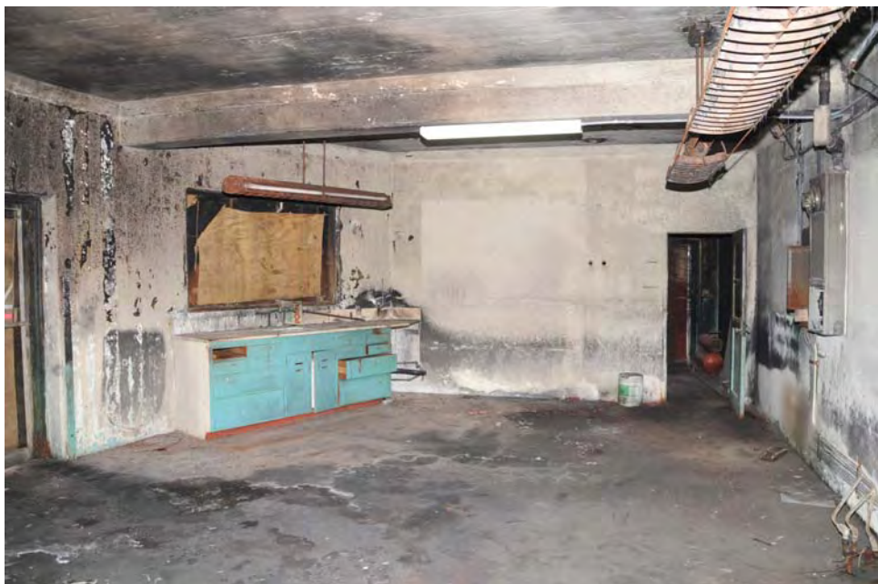
E-19 General view of the interior of the administration building, illustrating generally good condition of the concrete surfaces.
