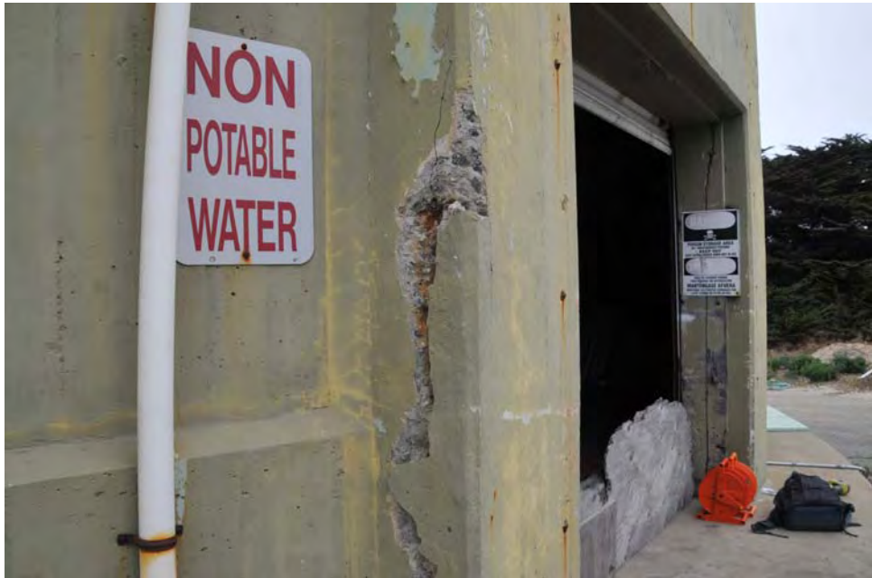
E-12 View of the primary rollup door, illustrating a large spall and random corrosion on the reinforcing steel and adjacent concrete.
