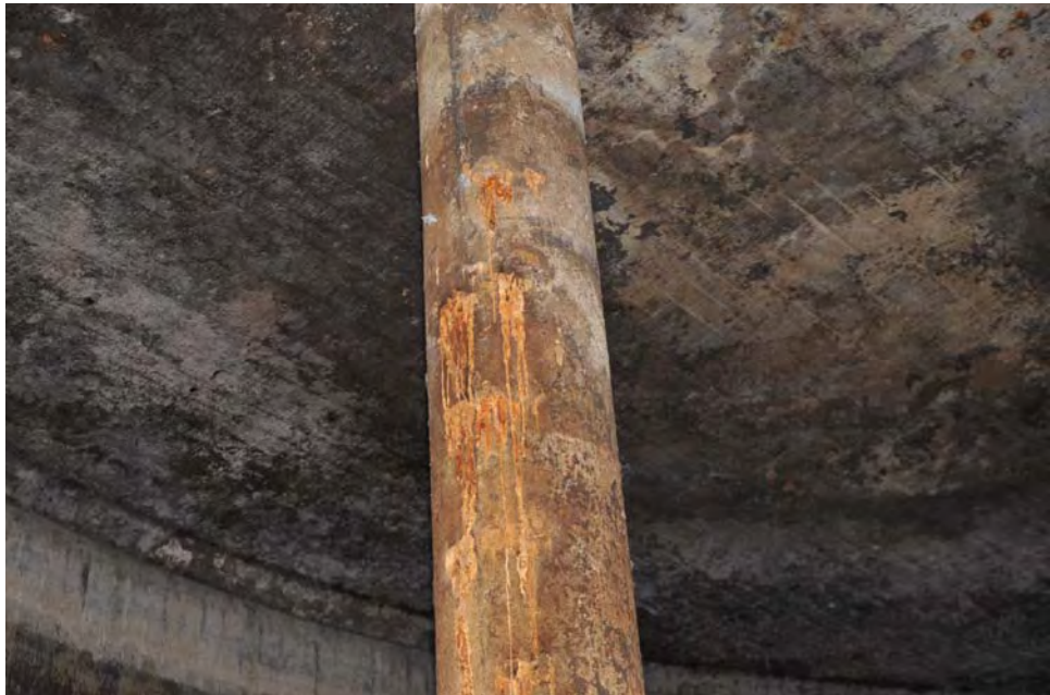
I-30 View of a column, illustrating moderate corrosion leaching from the concrete.
