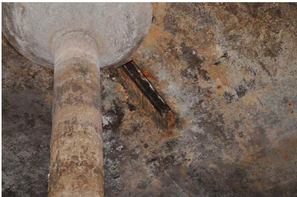
I-7 View of a roof penetration, illustrating corrosion and staining.
